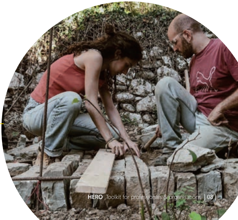
Workshop trainees during restoration works, Epirus, Greece.
