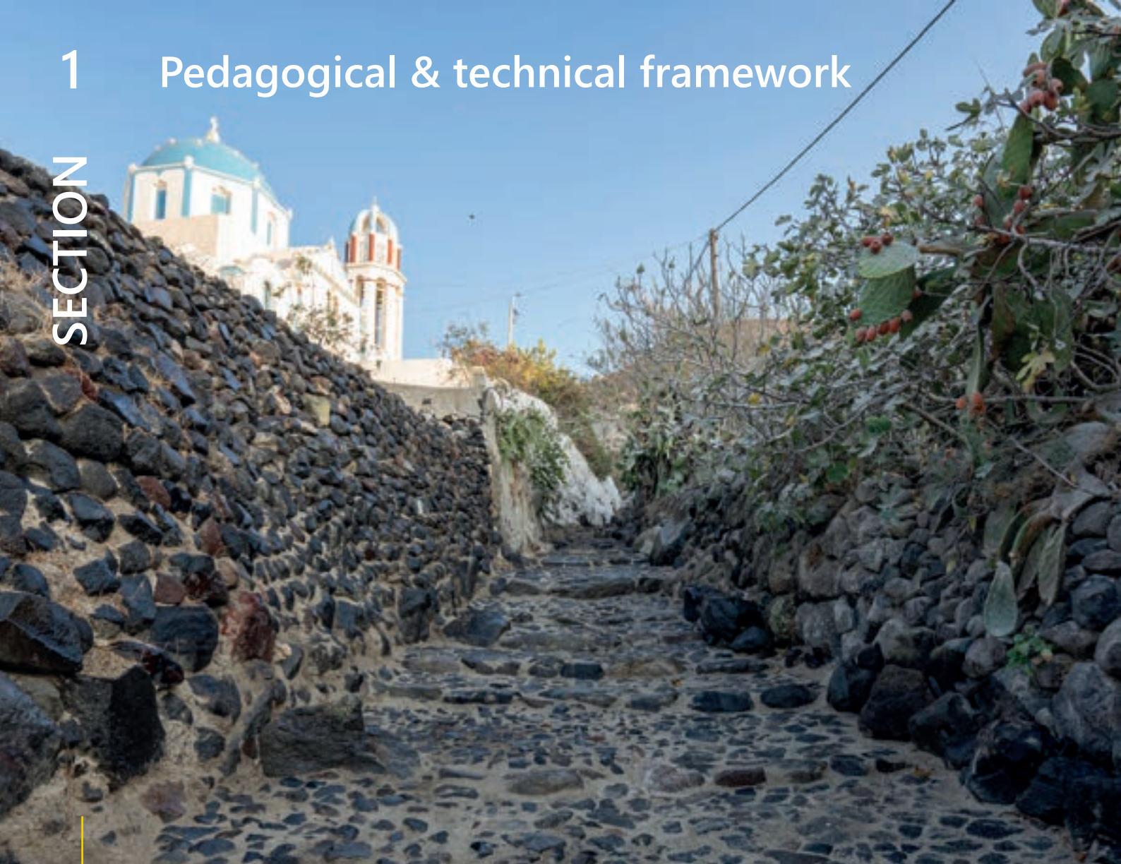
Drystone pathway and lateral walls made of volcanic stones in Cyclades, Greece.
