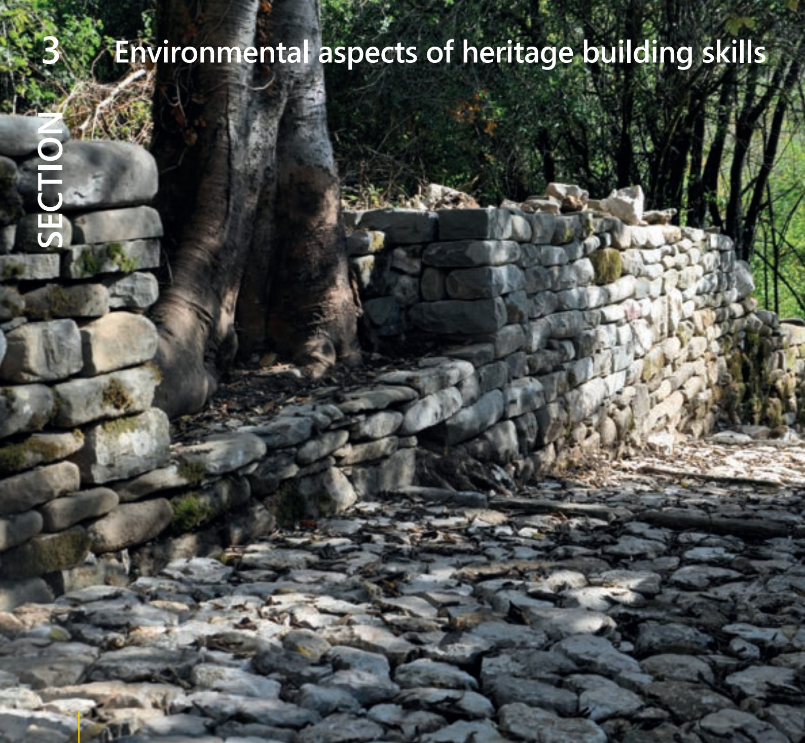
A drystone pathway and lateral walls interwoven with local trees, Epirus, Greece.
