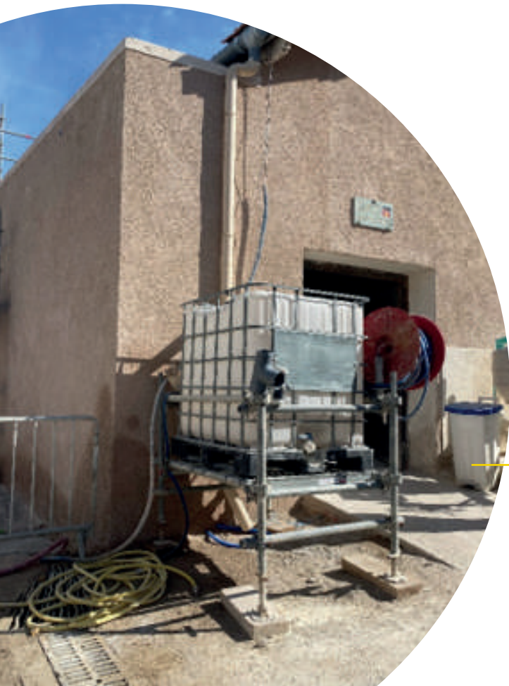
Example of a water tank collecting rainwaters for cleaning tolls Marseille, France
