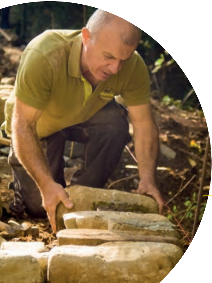
A stone mason placing the corner stones of a cobblestone, Epirus, Greece.
